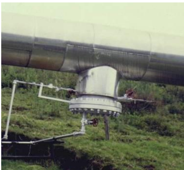
Figure 3.14 : Condensate collection drain pot (CCDP)
