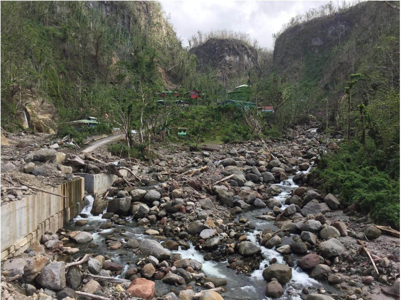
Figure 1.3 : The devastation caused by Hurricane Maria – Roseau Valley (taken in November 2017)
