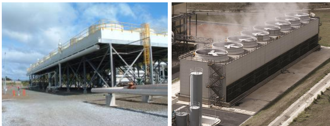
Figure 3.19 : Air cooling for 9MW binary plant (left). Evaporative cooling tower – only 1-2 cells likely required for Dominica project (right)
