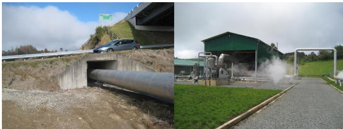
Figure 3.6 : Examples of a reinjection line culvert underneath a road (left) and a u-bend in a reinjection line (right)
