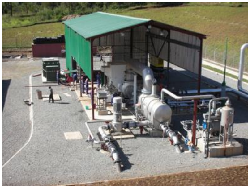
Figure 3.16 : Condensing Steam Turbine (Source: GDA - http://www.gdareno.com )
