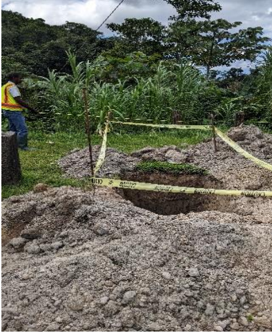
Figure 43. Trafalgar Power Station
