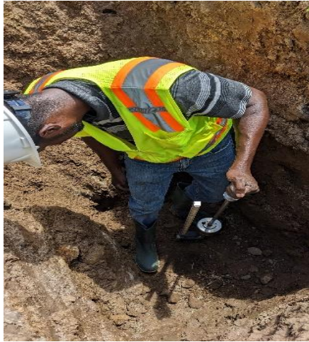
Figure 45. Fond Cole Power Station
