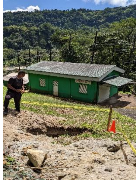
Figure 40. Padu Power Station
