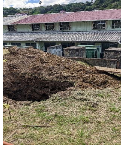
Figure 46. Fond Cole Power Station
